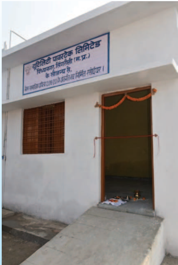
Construction of kitchen room with shades for school
